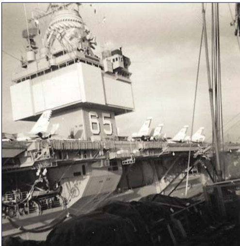
Figure 4: USS ENTERPRISE takes on fuel from KASKASKIA during UNREP in the Mediterranean March 1963.
